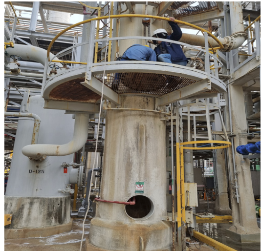
Fig. 4. Installation of the Gas Detector
