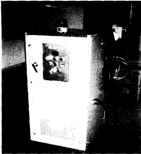
Figure 2. Gas vent box
