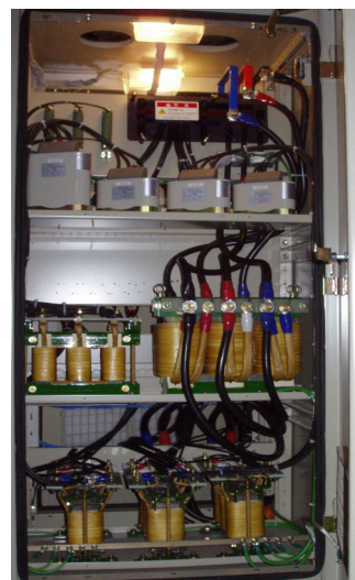
[Fig. 3] The designed passive filter
