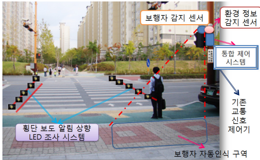
[Fig. 3] Assistive pedestrian safety measures the actual configuration of the system
