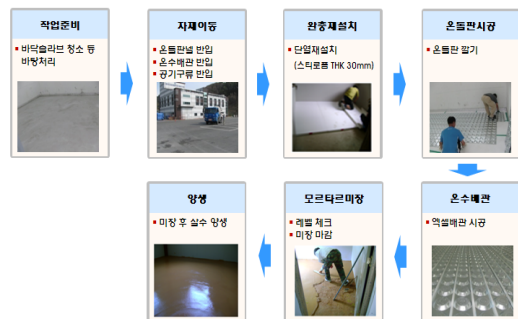
[Fig. 3] Ondol of floor heating work procedure
