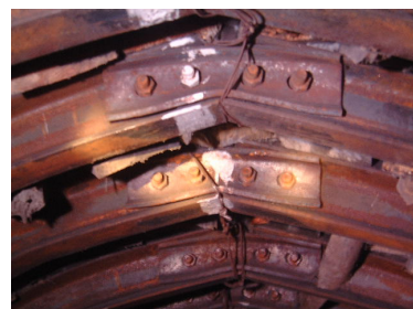
[Fig. 4] Photograph for bending of tunnel support
