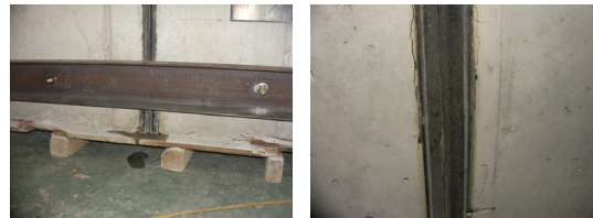
(a) 누수 (a) Water leak (b) 균열(실험체 B) (b) Crack(Specimen B)
