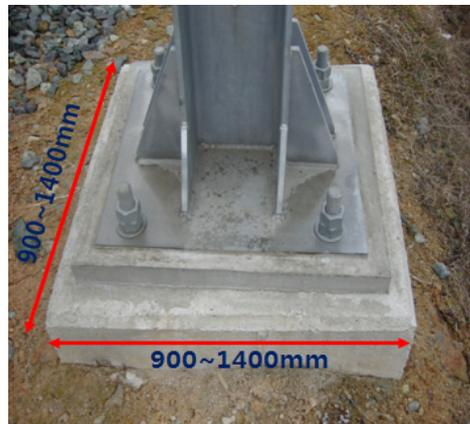
[Fig. 2] Rectangular concrete foundation for railway electric pole
