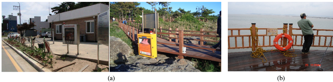
[Fig. 7] Rescue facility (a) Improper placement (b) Neglect of maintenance
