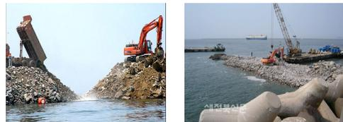
[Fig. 4] Traditional Embankment Technology With Riprap
