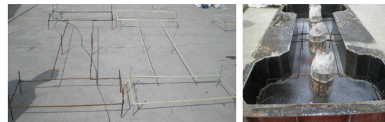
(a) GFRP(left) and Steel rebar(right) (b) Casting mould [Fig. 7] Reinforcing bar and form work(R-CS, R-RG)
