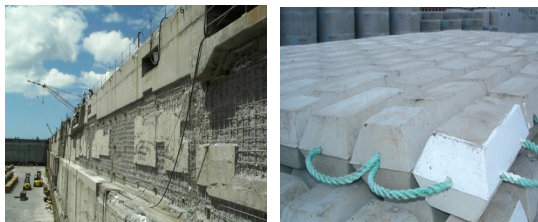
(a) Pearl harbor(U.S.A) (b) Concrete fleximat(Norway)
