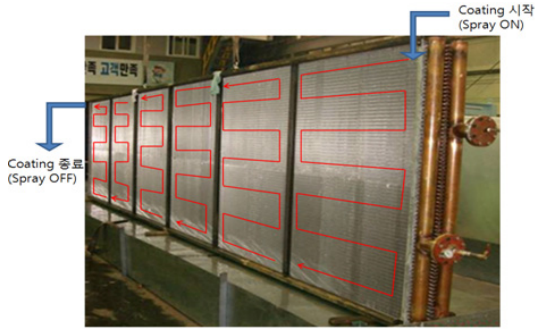
(a) Coating along block by block
