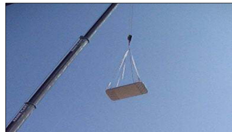
[Fig. 9] 65ft Lifting of Fuel Cell
