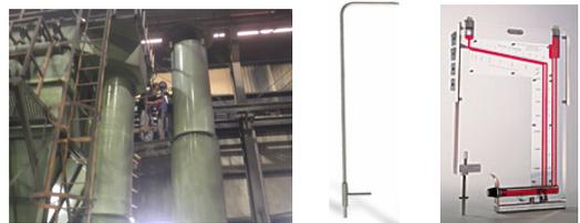
(a) Measurement of flow rate (b) Measurement equipment
