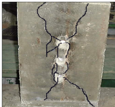
[Fig. 11] Split of concrete block
