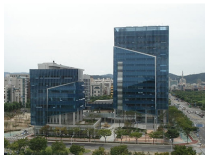
[Fig. 5] Overall view of project #2
