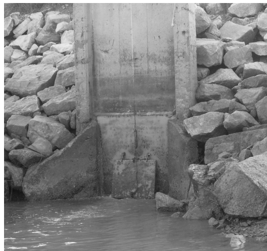
[Fig. 5] Present discharge gate
