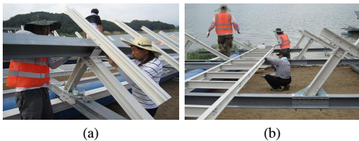
[Fig. 5] FRP structure assembly (a) Structure assembly (b) Foothold assembly
