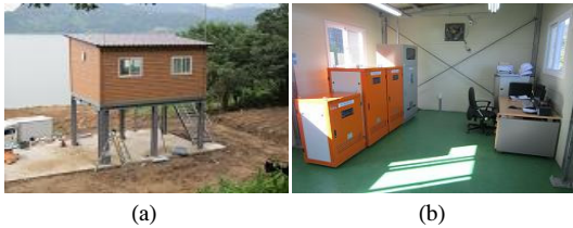
[Fig. 15] Construction of electric room (a) Newly constructed electric room (3m expansion) (b) Layout of electric room interior
