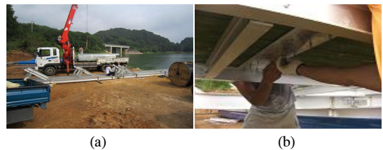
[Fig. 7] Aluminum structure assembly (a) Structure bolt assembly (b) Structure assembly
