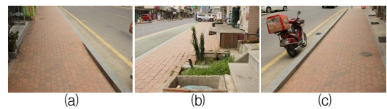
[Fig. 6] Sidewalk condition for pedestrian (a)Sloping sidewalk, (b)Uncovered sidewalk, (c)Raised spot of sidewalk
