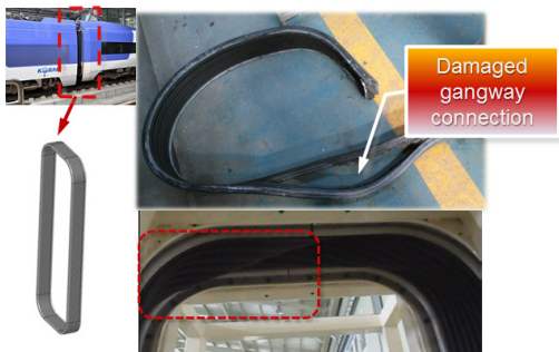
[Fig. 1] Damaged gangway connection of the articulated high speed railway vehicle
