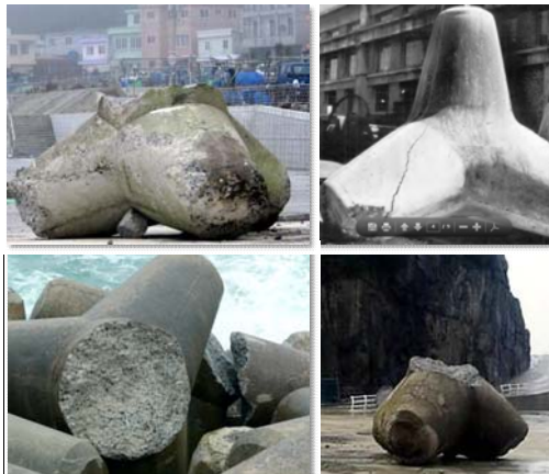
[Fig. 2] Failure state of tetrapod blocks
