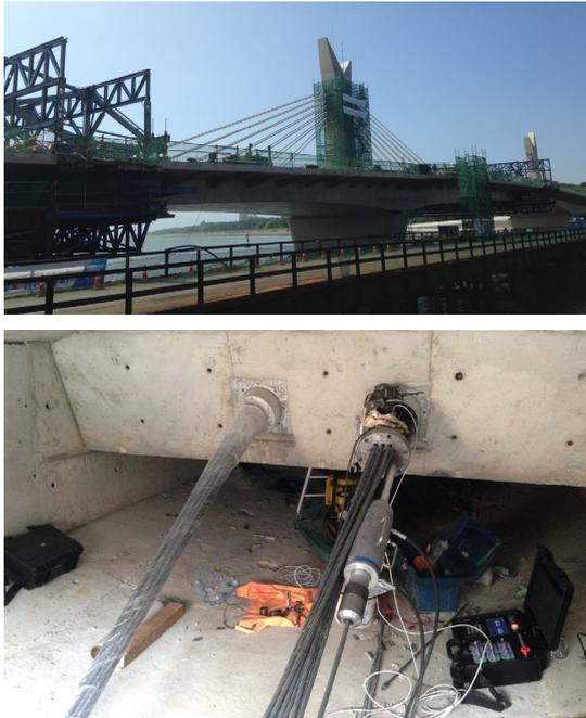
Fig. 15. 2<sup>nd</sup> Tain bridge and field application of electrical resistance iso-tensioning system
