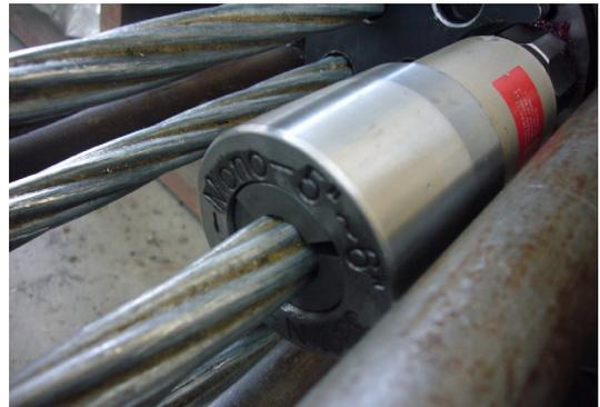
Fig. 9. Temporary wedging by rear block
